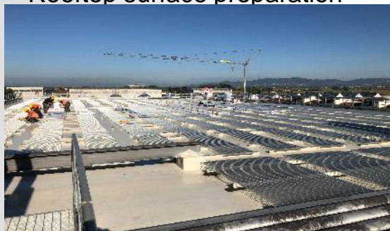
Substructure for panel installation
