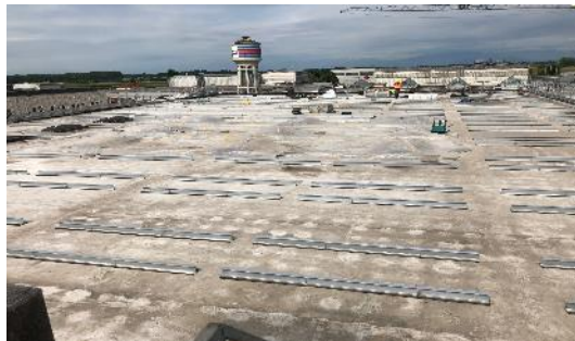
Beams for substructure
