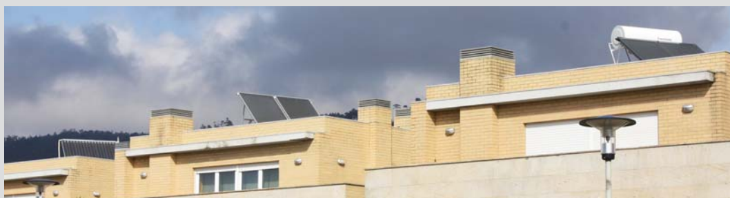
Figure 1: Example of three different installations. From left to right, forced circulation with evacuated tubes, forced circulation with flat plate collector and thermosiphon with flat plate collectors. Photo: J.Seco / ESTIF
